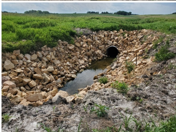
Completed photo of the fencing, armoring culverts and sensitive areas.
