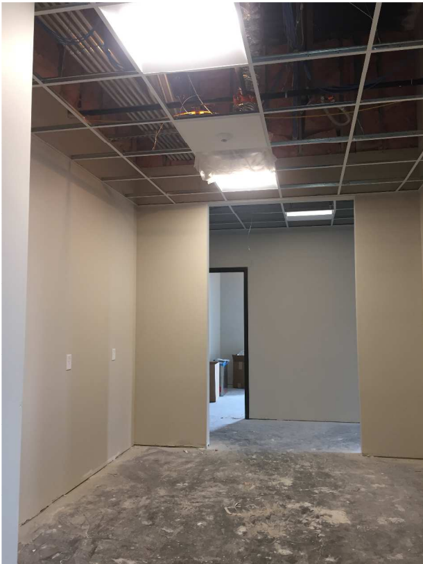
Second floor painting and ceiling grid were completed in the first few zone!
