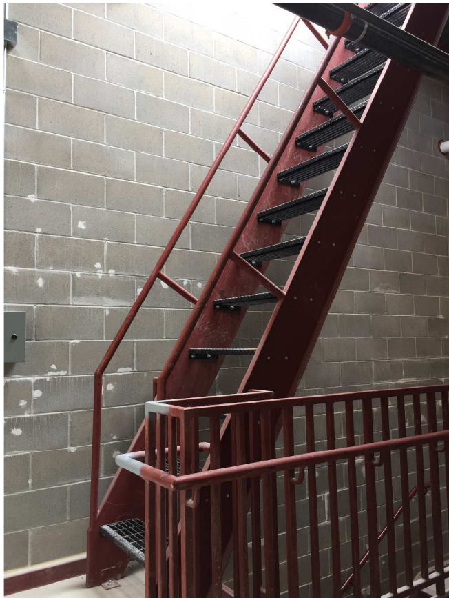
The steel ships ladder was installed making way for the painters to paint the stairwell! This ladder gives access to the roof
