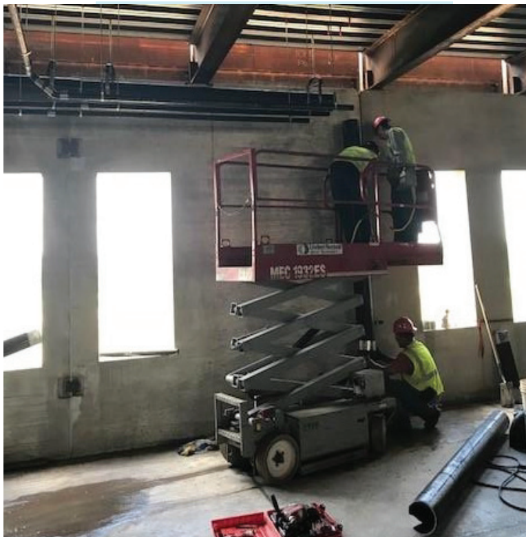
Rough-ins started to take off in Area A as well.
