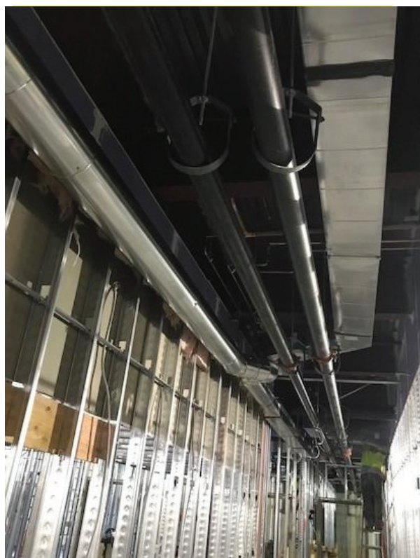
The MEP contractors continue to do rough-ins in the lower level.
