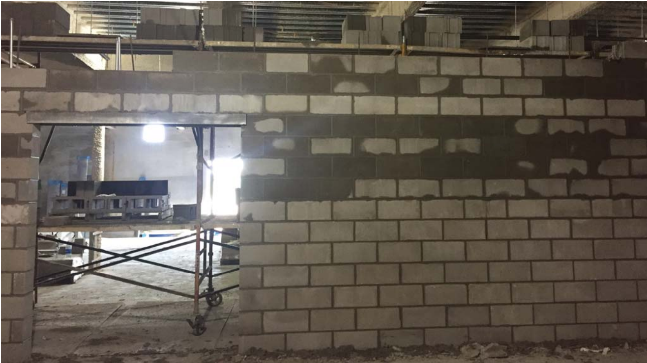
CMU structural walls are put up in Areas A and B.
