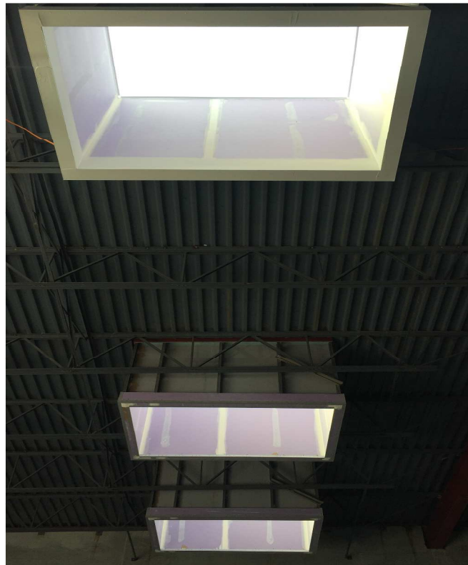
Skylights were installed in the Area B roof
