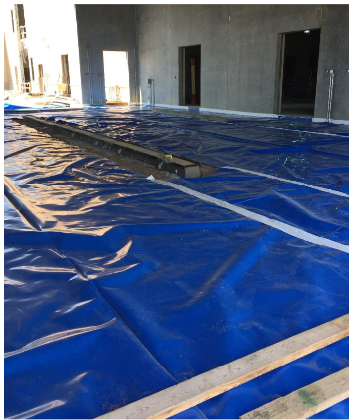
Northland Concrete prepared for their last big pour in the sallyport
