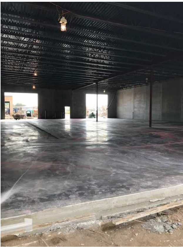
The floor of the LEC Garage was poured on Thursday
